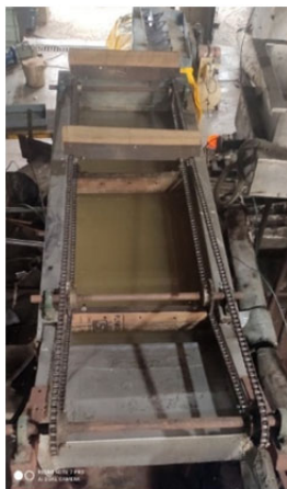
Sugarcane Juice clarifier
